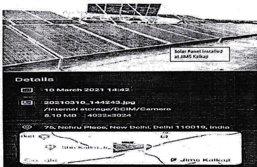
Solar panel installed at JIMS Kalkaji
